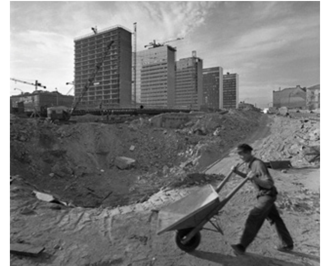
Figure 2: Residential buildings made way for modern inner-city office spaces during the city sanitation project. (Photo: Lennart af Petersen).
